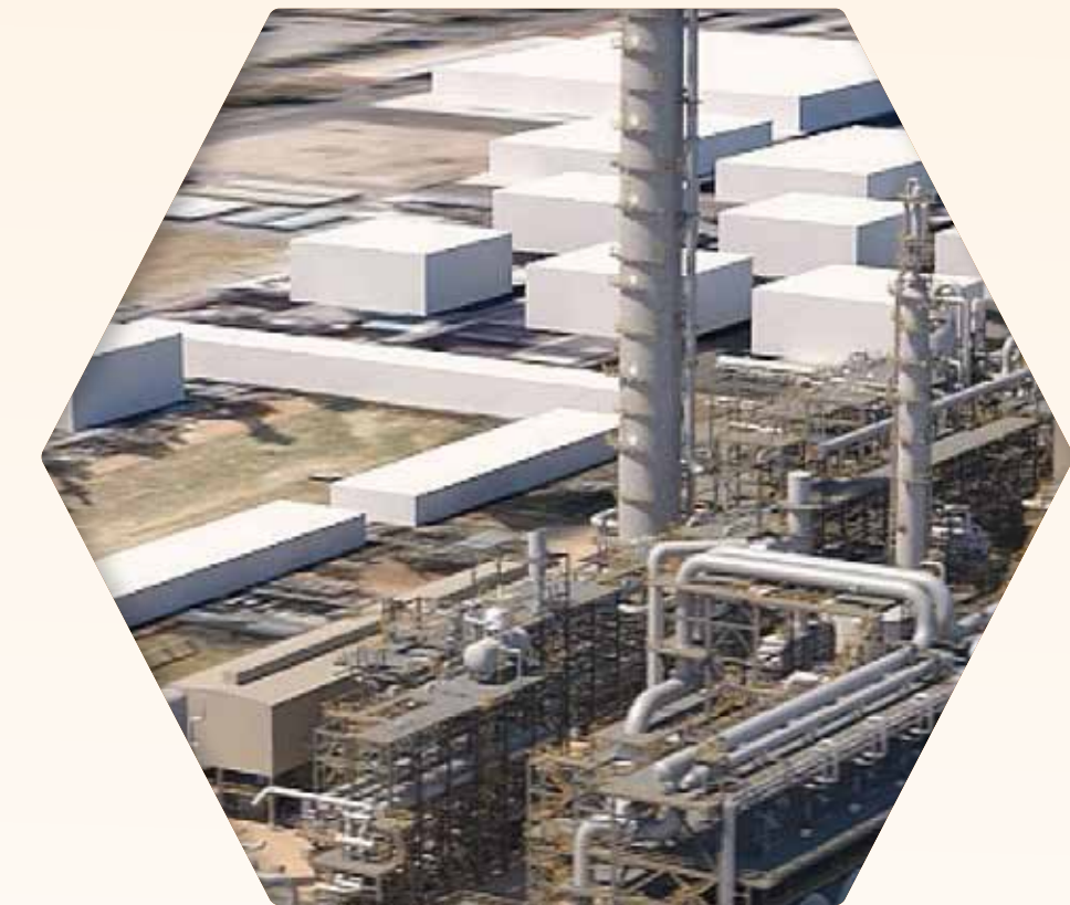
INEOS Project ONE: ethane gas cracker with the lowest carbon footprint in the world
