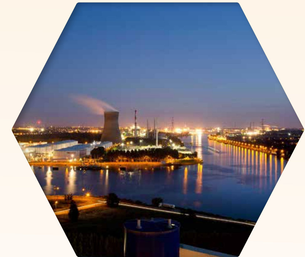
North-C-Methanol: production of green methanol based on hydrogen and captured CO 2 in Ghent port area
